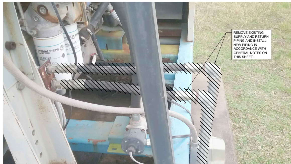
3 DIESEL FUEL SUPPLY & RETURN LINES C-02
